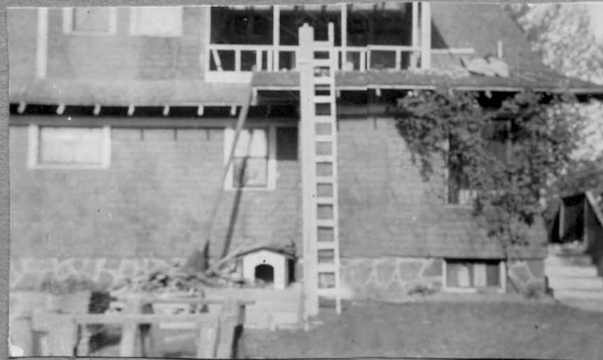
Back (Sleeping porch being added)
