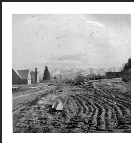
End of 31st Ave
