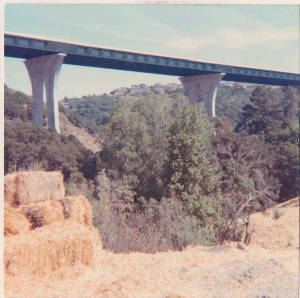
new bridge on new Skyline Freeway...
